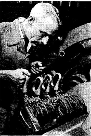
You had an arrangement in the laboratory when you reversed the direction of the current in the coil every  $180^\circ$  so that the forces continued to make the coil move in one direction. Such an arrangement for reversing the direction of the current is called a *commutator*. The conductors which make contact with the commutator are usually called the *brushes*.
